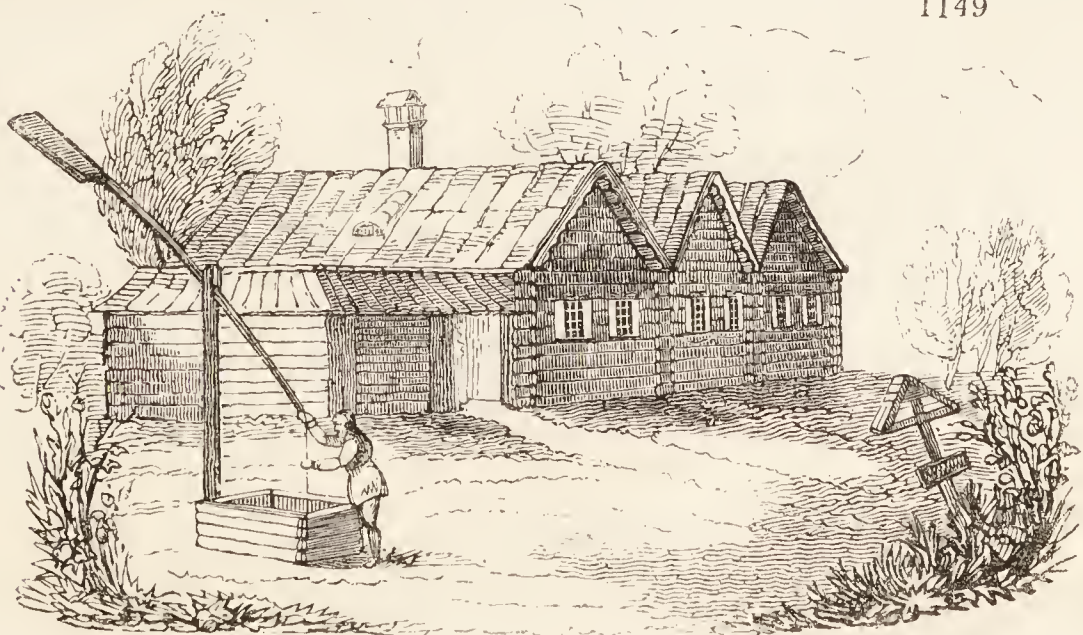
g b h a c e d f in 1832. The buildings consist of a dwelling-house ( a ), with a detached kitchen ( b ), a brewery ( c ), a distillery ( d ), a machine for raising water to supply both ( e ), a corn-mill ( f ), sheds for feeding cattle ( g ), an ice-house ( h ), in which ice is kept above ground by means of thick double walls and doors; and large barns, a threshing-machine, coach-house, stabling and all other offices, including a carpenter's shop and house, blacksmith's shop and house, bailiff's house, &c. Besides these there is a small colony of cottages for the common labourers. These cottages are generally of the kind called log houses, and, with their draw-wells attached, present the appearance of fig. 1149. The Germans who are settled in Poland, as agricul-
